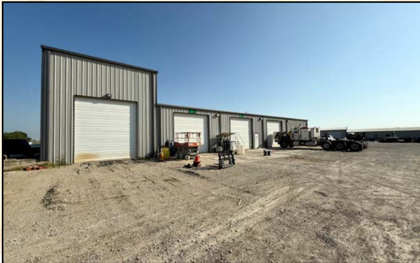
5901 New Addition to the Warehouse adding an additional 1,875 sq ft. to building 2
