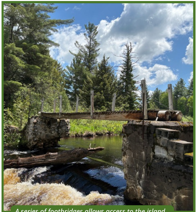
A series of footbridges allows access to the island and the western shore of the river above the falls.
